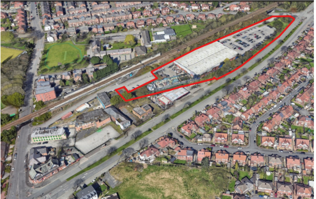
Aerial view with the application site edged in red
