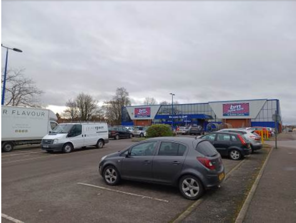
View south across car park towards existing retail store
